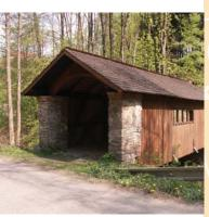
The valuable sight is also a covered beam bridge over river Nedvědička in a village Pernštejn. It is 4 metres wide and 12 metres long. It has got four windows in side walls and is covered with shingle. It was mentioned for the first time in 1864, it was renovated in 1933. It went through an extensive renovation in 2004. The four brick corner pillars are the speciality of this bridge.
