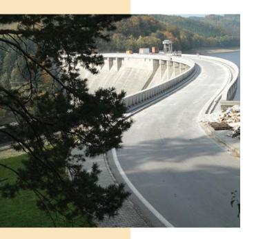
The mighty construction above Vír totally changed the local landscape and flooded the exquisite valley around Chudobín. The preparation of foundations of the concrete dam started in 1949. This dam is now the third highest dam in our country (76,5 m). The funicular from Bystřice transported the material to the building site. The whole construction ended in 1957.
