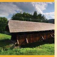
The shingle covered wooden bridge over river Svratka in Černvír is from 1718 and should be the oldest in Moravia. It is 32 m long and 2,6 m wide, it has got a hanging construction, building material is fir and partly oak. It was pulled down by flood in 1761. It was used till 1954. It was carefuly repaired in 1971 the shingle was put on in 1996. The replacement of the supporting beams took place recently. The bridge is even displayed on post stamps.
